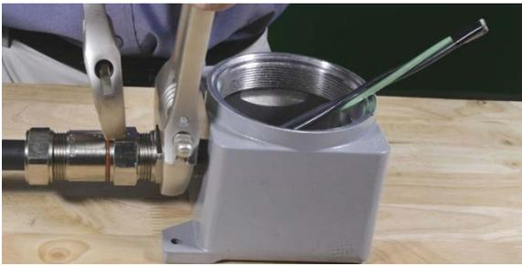
Once the nut is hand tight, place a wrench on the hub nut and the barrel nut. Fully tighten the hub nut to the connector in this fashion.
