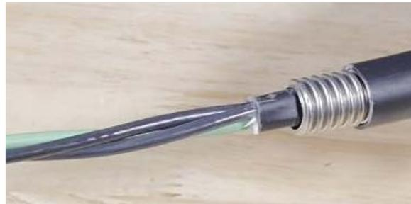
Remove all but 1/2 inch [1.3cm], measured from the end of the armor, of the cable core's jacket and binders. This will allow the sealant to be injected into the spaces between the cable's components, blocking the flow of gasses in an emergency.
