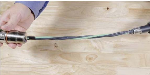
Once reaching the exposed armor, rotate the connector by hand while applying gentle pressure. Continue rotating the connector in this manner until it is hand tight.
