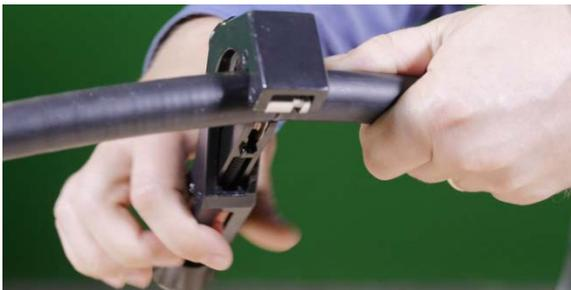
Once cut, the Dekaflex® armor can be removed, exposing the cable's core. Be careful not to cut too deeply, as this could result in damage to the core.
