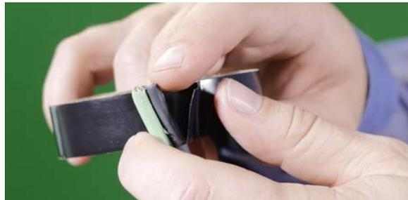
To keep the conductors bunched and aid with conductor installation, wrap the loose ends of the conductors in electrical tape.
