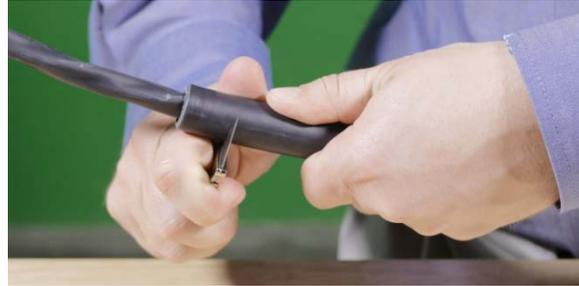
While removing the outer jacket, if too much armor was exposed, simply cut away a small portion of the armor to correct the issue. If too little was exposed, remove more of the outer jacket. Removing an excessive length of the outer jacket is not recommended and should be avoided. Failure to remove the correct amount of outer jacket could result in a poor-fitting connector and faulty installation.
