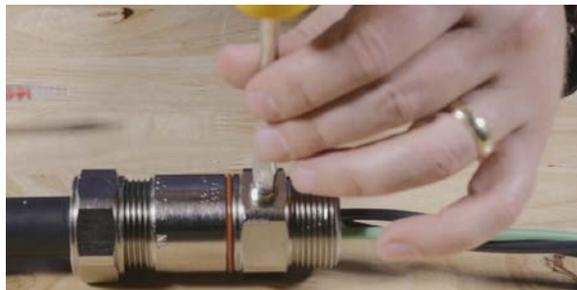
Now, place the self-mixing applicator tip in the inspection port or the end of the barrel and inject the sealant into the connector until the cavity is filled.
