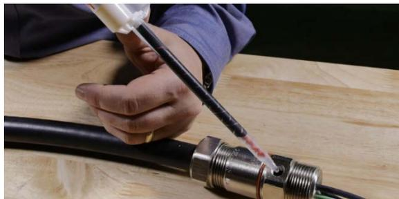
Allow a few seconds for the sealant to fill the voids in the cable, and add more sealant as needed. Once completely filled, the inspection port covers should be replaced if they were previously removed.
