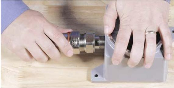
Once the hub is hand-tight, use a wrench placed around the connector barrel nut to tighten the hub to the enclosure. When the hub is tight, place a second wrench around the hub nut and loosen it.
